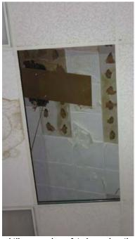
Photo 11 – Original tiles posed a safety hazard as they fall and displace the ceiling below
