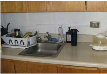
Photo 14 – Lack of GFCI outlet adjacent to water source
