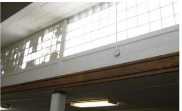
Photo 6 – Clerestories have been partially painted over to address glare issues within repurposed spaces
