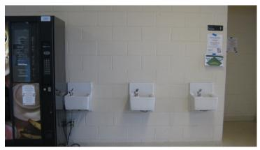
Photo 12 – Lack of dual-height drinking fountains; exposed pipes
