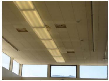
Photo 8 – Water damaged/missing ceiling tiles
