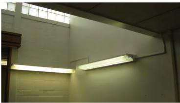
Photo 7 – Insufficient infrastructure and CMU wall construction has resulted in unsighly wiring around most classrooms
