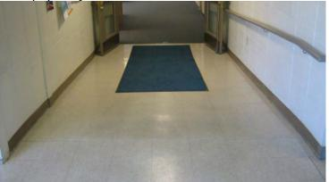
Photo 17A - Ramp in corridor (along egress path) lacks level surface prior to placement of doors
