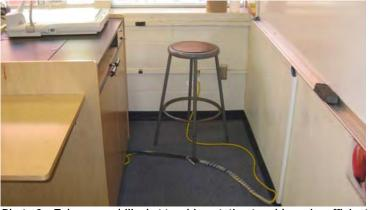
Photo 9 – Telecom umbilical at teaching station to address insufficient infrastructure
