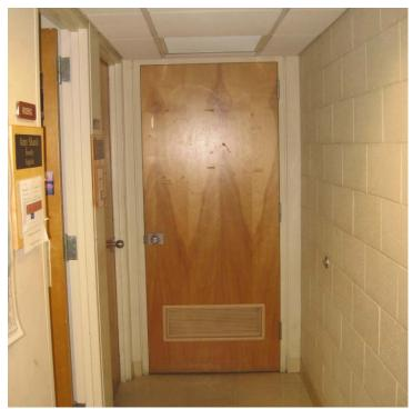
Photo 2 – Door does not have adequate accessibility clearances on push-pull side
