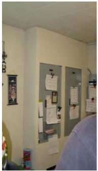
Photo 12 – Lack of tackable wall surface results in electrical panels acting as bulletin boards.
