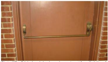
Photo 18B - Original panic hardware does not meet force limiations for accessibility requirements
