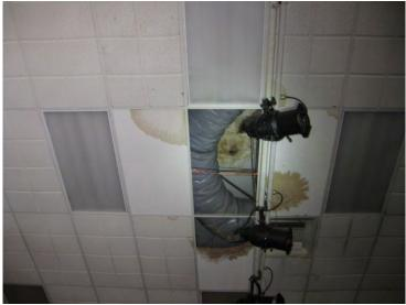
Photo 15B – Evidence of previous water damage on ceiling tiles
